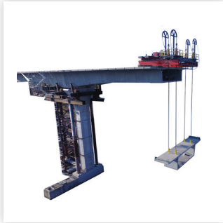
Cantilever Segmental Bridge Lift System
